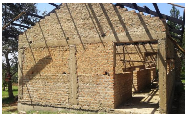
Outcomes: Construction of Nyankwanzi HC III new maternity ward
